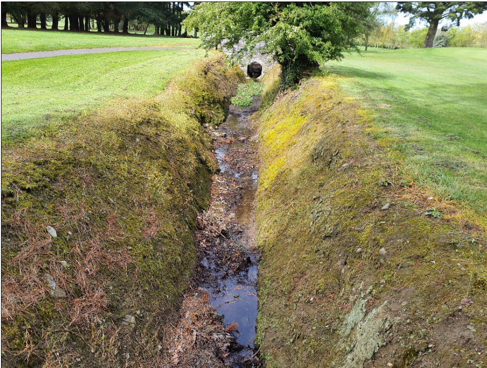
Figure 12 Drainage ditch with sprayed banks
